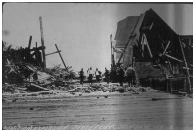
Photo of the rail yard terminal building after the explosion
