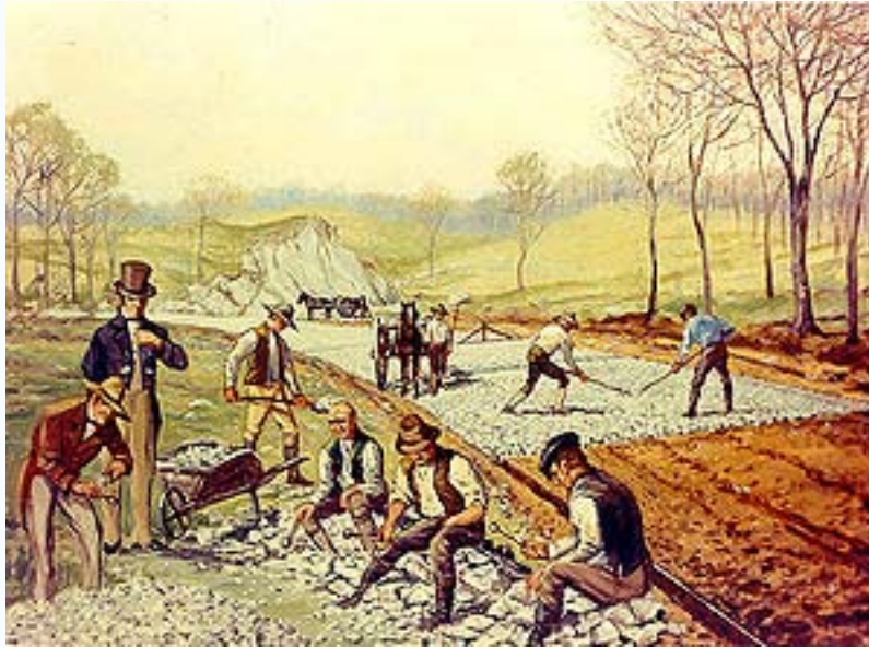
Workers laying a section of the new Macadam road
