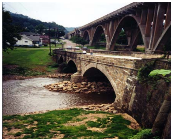
The Old and new Blaine Bridge in Ohio
