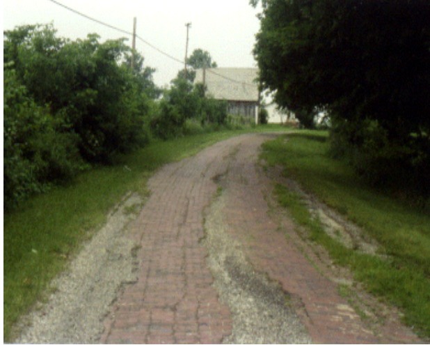
A remaining section of the original road in Guernsey County in Ohio
