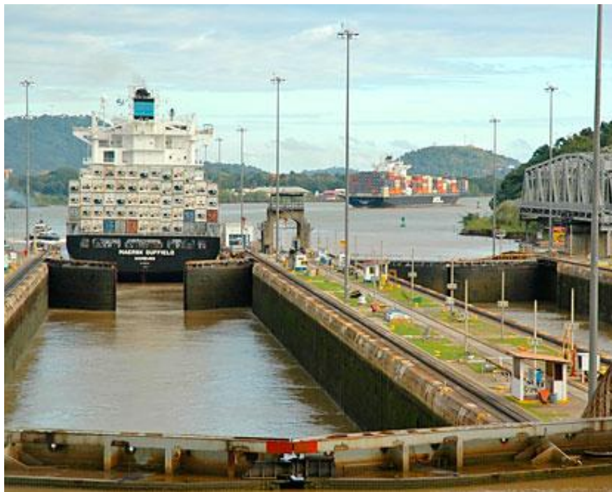
A photo of a canal lock in use today. Note how narrow it is and because of this plans are under way to widen the canal so the newer, larger cargo ships can pass through easier. Cruise ships actually overhand the sides of the locks! See the next two photographs.
