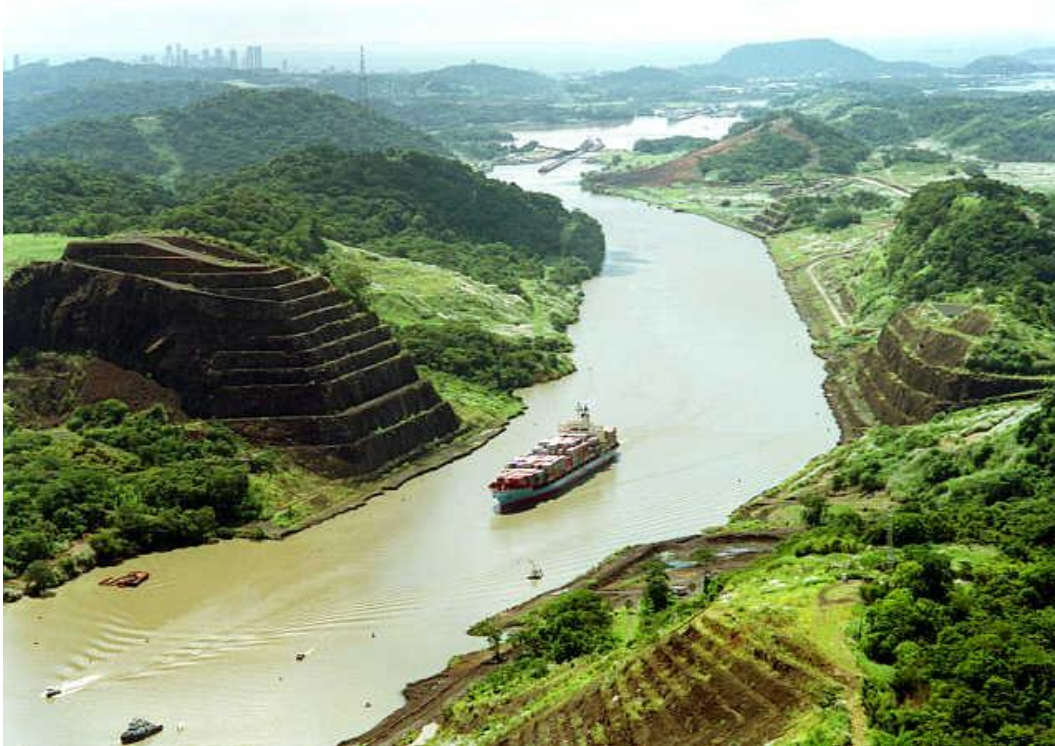
An aerial view of a Maersk Line cargo ship in the canal
