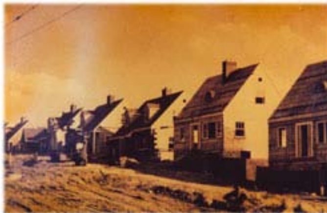
Levitt built 30 to 40 houses a day using an assembly line technique
